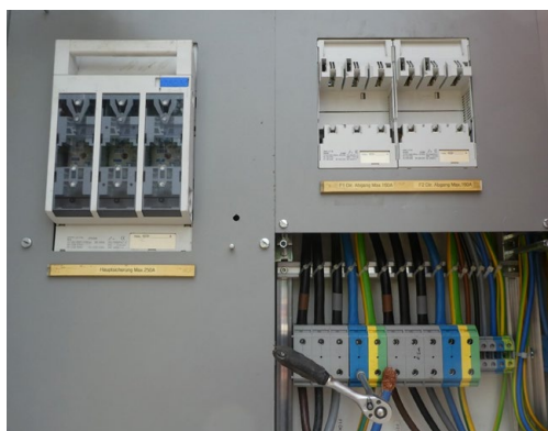
Figure 16: Tableau de chantier (source: ESTI)
